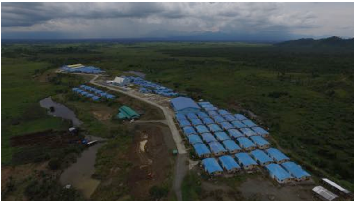
Photo 1 The Iglesia Ni Cristo resettlement project located in Alang-alang, Leyte, which consists of housing units, eco-farm and other livelihood facilities built for the displaced victims of Super Typhoon Yolanda (Haiyan).
