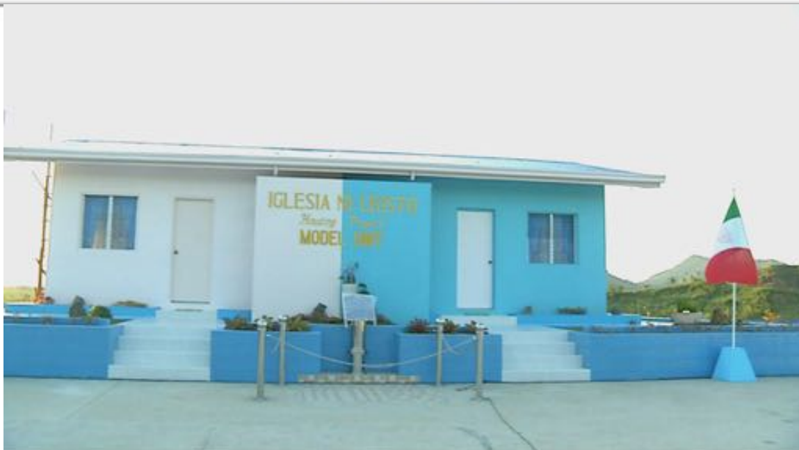
Photo 2 Up close, a model of the housing units in the Alang-alang settlement in Tacloban.
